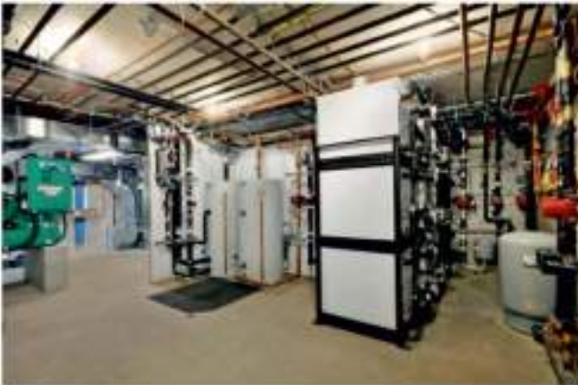
Pool Plumbing and Installation
